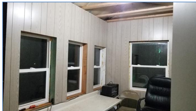
The crow's nest renovation is nearing completion!
